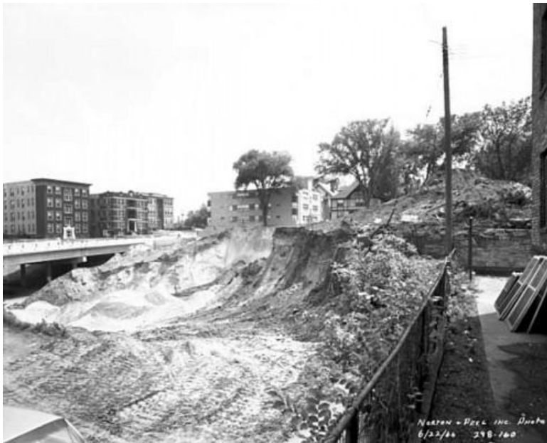
I-94 Construction through Rondo, 1966 Photo Source: MN Historical Society
