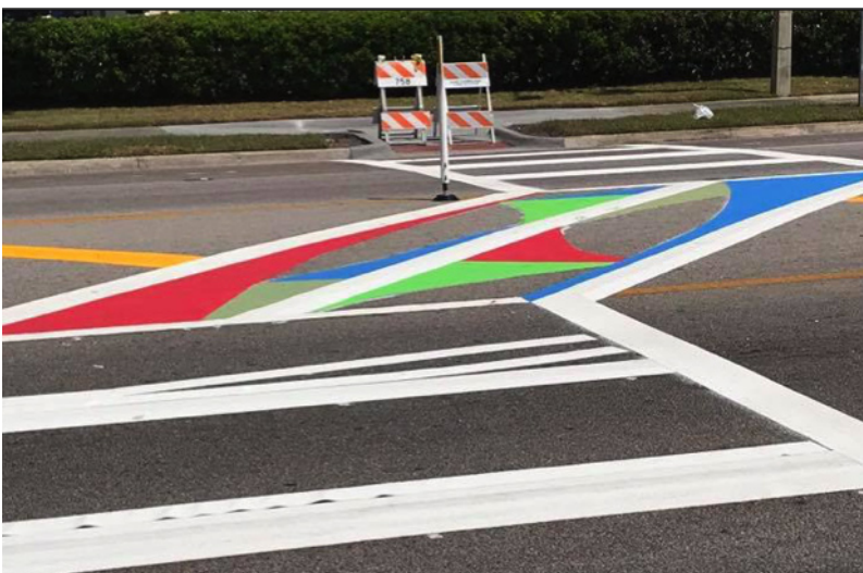
Workers used paint and tape to install a new mid-block crossing on Curry Ford Road.
