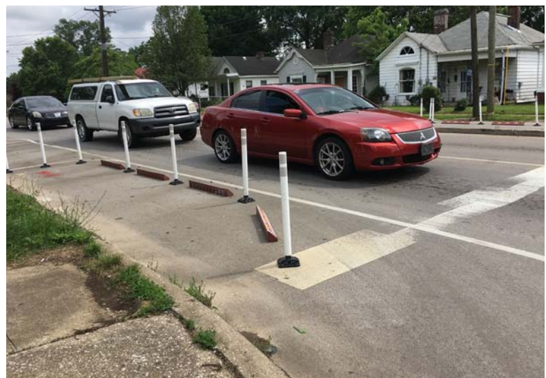
Lexington's redesign of Bryan and East Loudon Avenues included bump outs and a protected mid-block crossing using temporary vertical posts.
