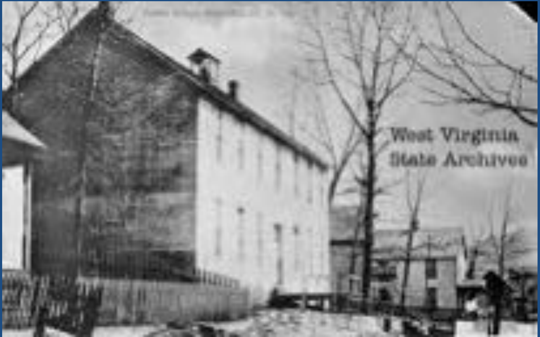
Hendricks High School and surrounding neighborhood (early 1900s)
