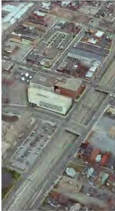
Aerial View of Existing Inner Loop Expressway Section Between Monroe Avenue and Charlotte Street
