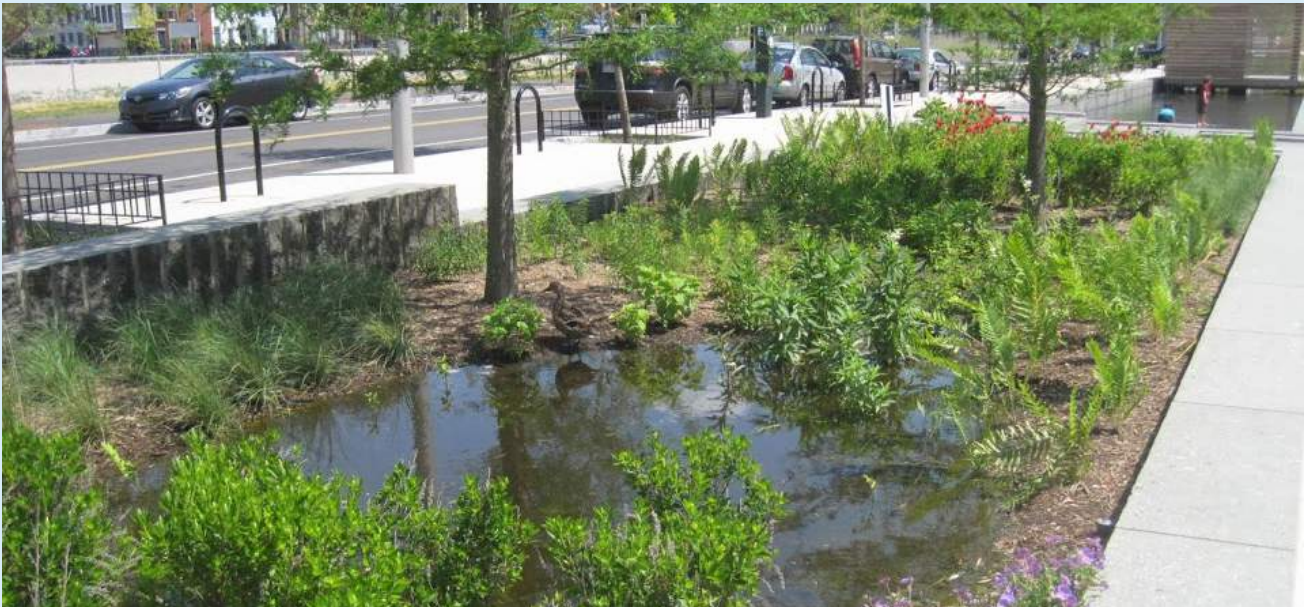
Healthy Communities Grant Program funding can be used to install green infrastructure, like rain gardens, to manage stormwater.
