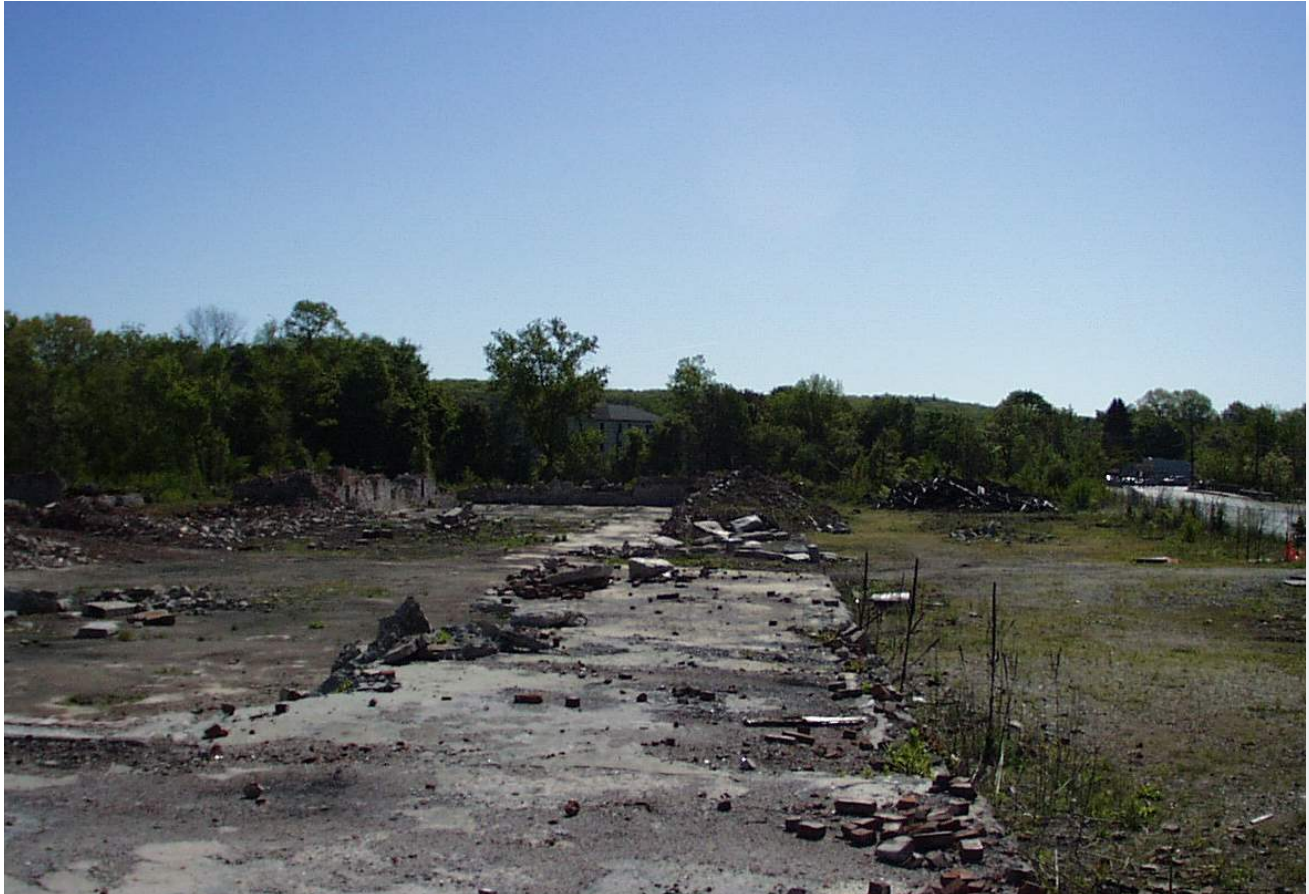
Pre-cleanup Brownfield site of Fisherville Mills in Grafton, Massachusetts. Photo: Massachusetts Department of Environmental Protection
