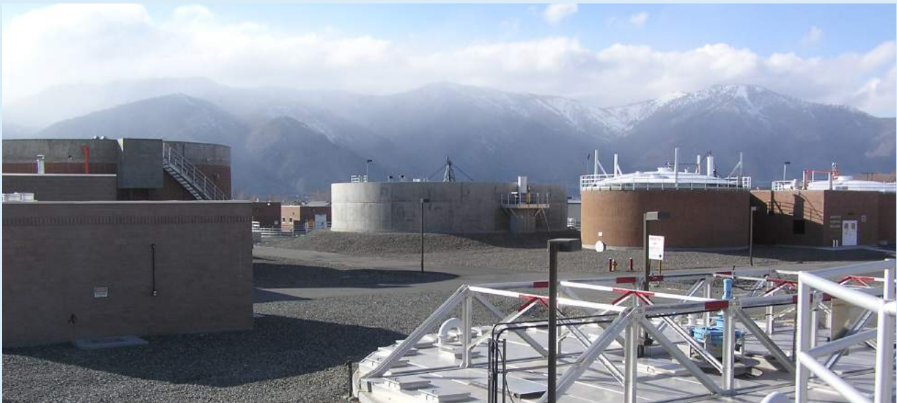
Wastewater infrastructure funded by Nevada's State Revolving Fund
