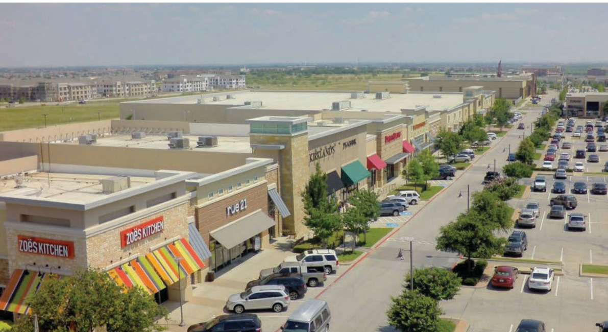
Retail area in AllianceTexas. (Credit: Heritage Homes )
